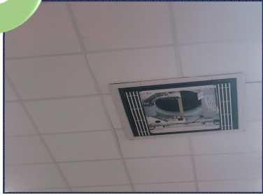
A/C ROOF INSULATION
